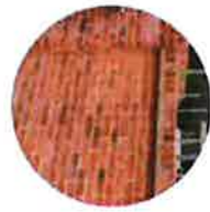
Brickwork - Hampton Rural Board by Fethers
